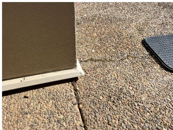
Figures 5 and 6: Figures 5 and 6 illustrate separation and displacement along the slab edge, consistent with differential movement between the slab and adjacent ground. These conditions indicate subgrade instability or loss of support at the slab perimeter.
