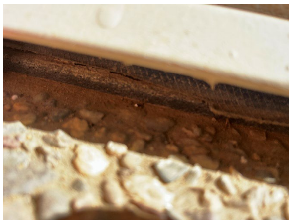
Figures 5 and 6: Figures 5 and 6 illustrate separation and displacement along the slab edge, consistent with differential movement between the slab and adjacent ground. These conditions indicate subgrade instability or loss of support at the slab perimeter.
