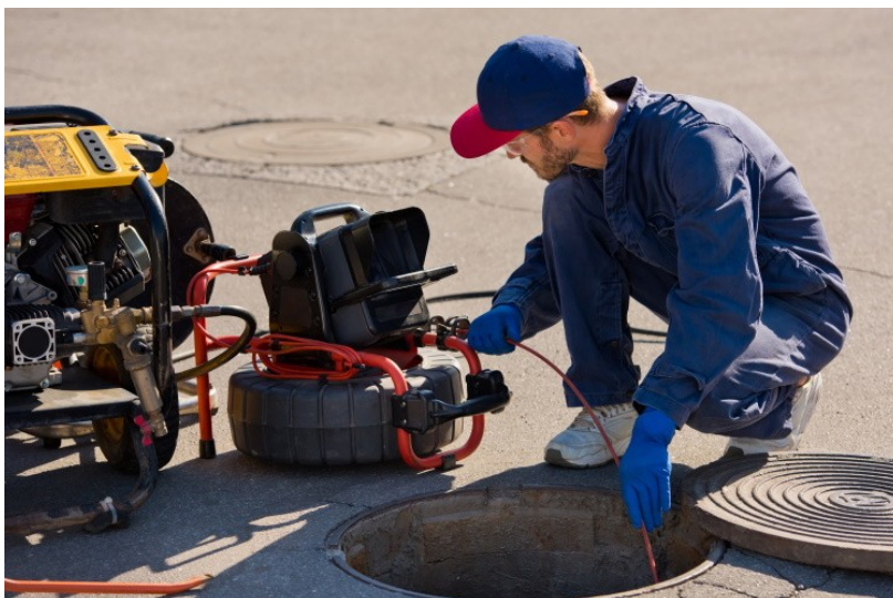
Figure 3 | Deploying a camera into a maintenance hole. Access is still the precondition; the camera does not create an entry point.
