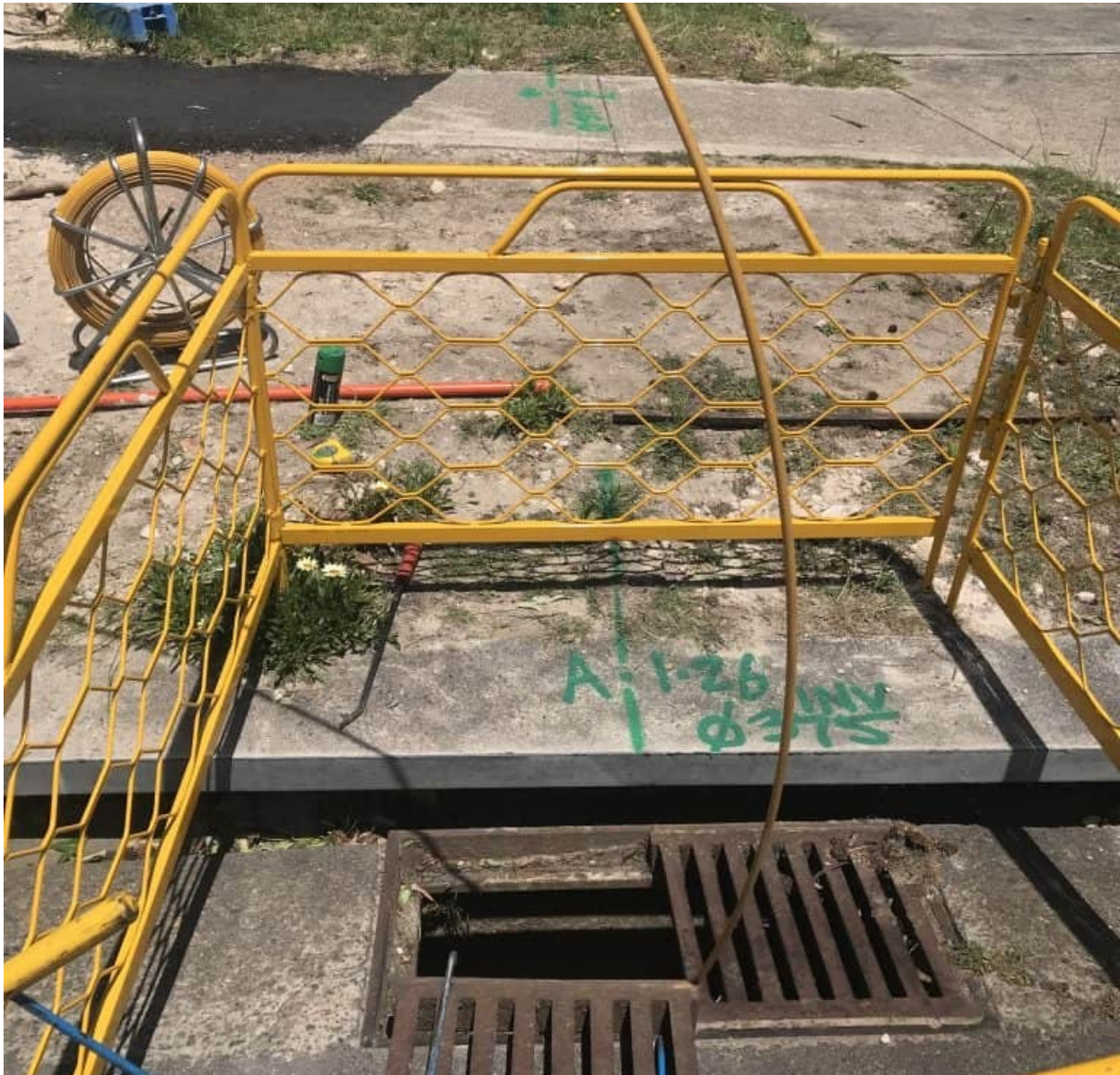
Figure 7 | An open, serviceable pit, with the trace marked and annotated on the surface. This is what a QL-B result looks like on the ground, and it depends entirely on the lid having come off.
