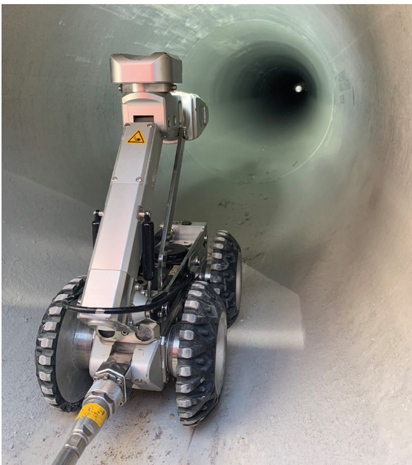
Figure 4 | A crawler unit in the line. Internal inspection converts guesswork about junctions and connections into measured fact.
