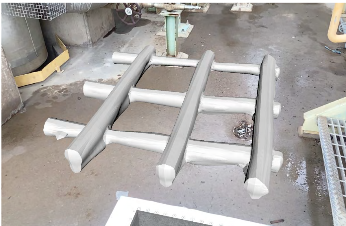
Figure 11: 3D visualisation of the scan data procured for Figure 9 above, confirming the overlap of the bars, including the placement of the east-to-west bars over the north-to-south bars (alternate angle)
